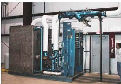
**STRAINERS WITH AUTOMATIC BLOWDOWN:** This OE type system has a Stainless Steel coldwell and automated strainers. Pressure differential is monitored across the strainers. When the preset trip pressure is reached, automated valves open and flush the strainers for a preset period of time.
