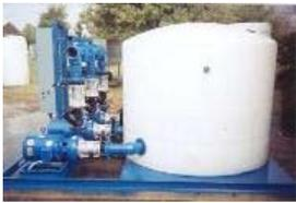
**POLY TANKS:** Shown at left is a packaged pump and control unit with a high density polyethylene coldwell. The tank is isolated from piping stress with flexible connections. Tank sizes range from 150 GPM to 5000 GPM.
