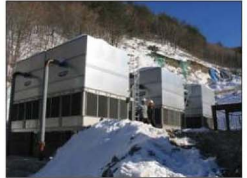
A Closed-loop Evaporative Cooler System
